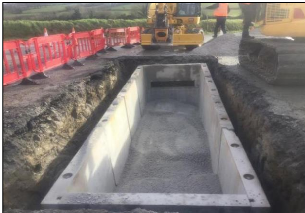
Plate 2-4 Pre-cast Joint Bay installation
