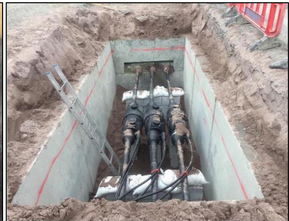
Plate 2-5 Joint Bay with Cable Jointing
